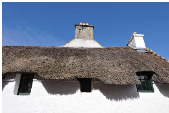
One of the most photographed roofs in Scotland, but now it's 33 years old and leaking
